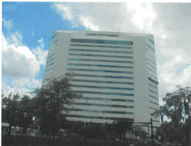
Office building north of campus
